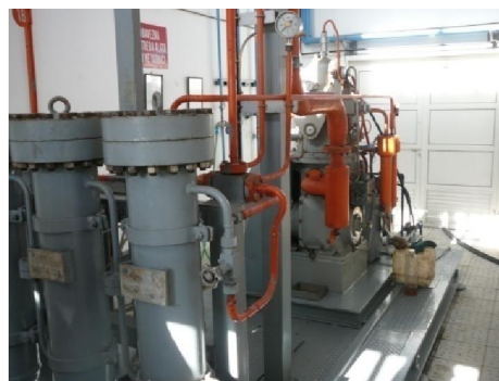
Picture 2. Batteries with calcium carbide
