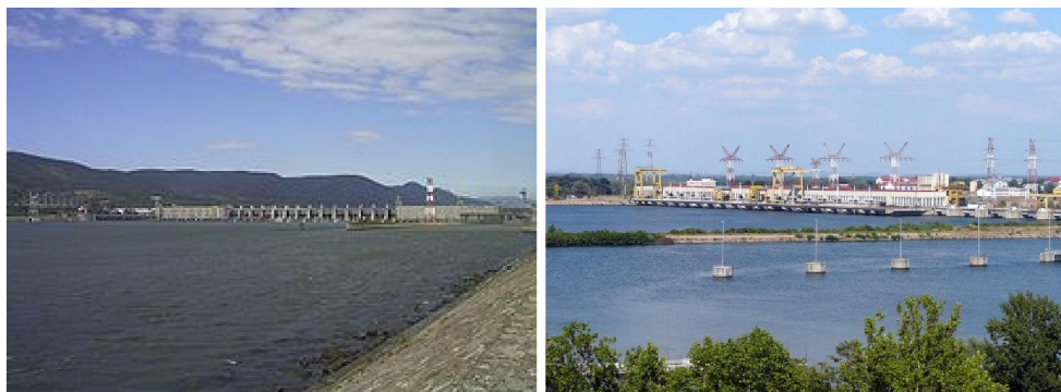
Figure 3. Hydroelectric power plants "Iron Gate I"(left) and "Iron Gate II"(right)
