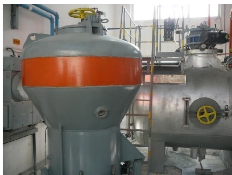
Picture 1. Developer's generator
