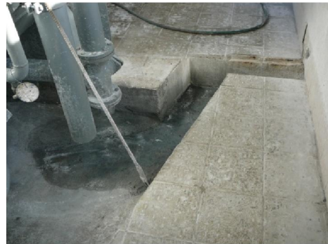
Picture 6. Canal for discharge of lime sludge from developer
