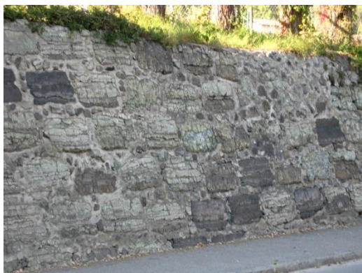
Figure 1. Wall built from the blocks of 19 th century blast furnace slag from Prevalje
