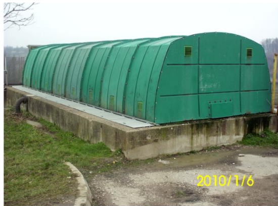
Figure 1. BIO-DISK plant for wastewater treatment at the mine Dubrave
