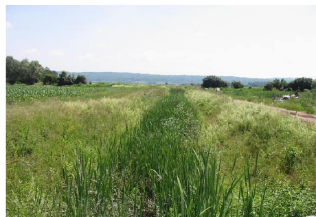
Figure 3. The current irrigation canal
