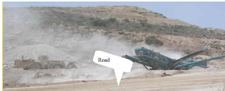
Picture 2. Stone exploitation, mobile crushing and sieving, 'Brankovina' quarry.
