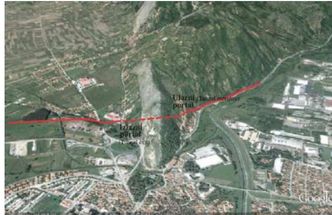
Figure 1. The tunnel route,, Sarlah " with entrance and exit portal
