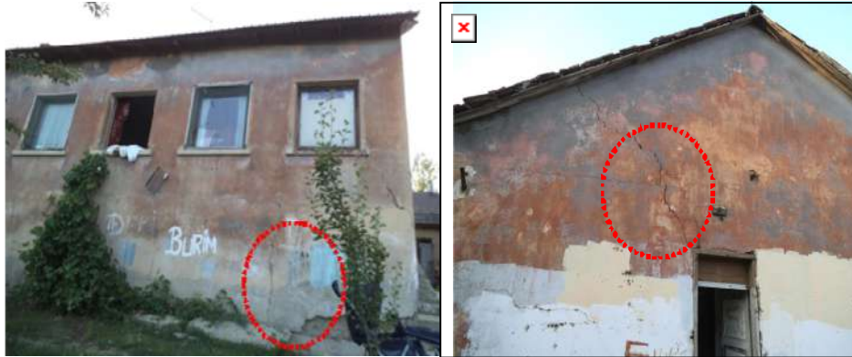
Figure 3. Fractures on front wall and side walls of house in Dositeja Obradovica 38
