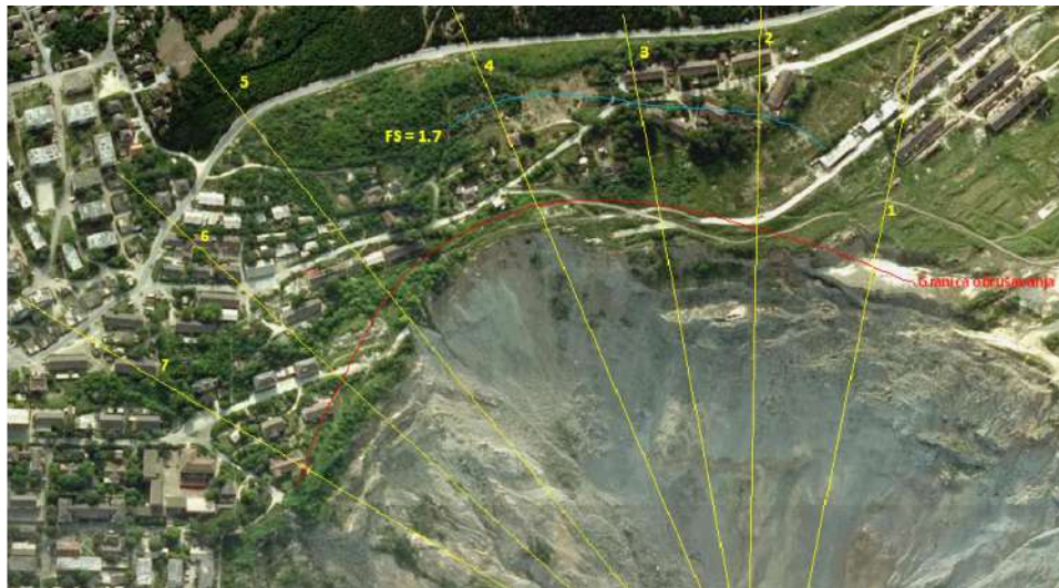
Figure 1. Orthophotograph of open pit slope and LC Sever with cross sections and influence zone boundary
