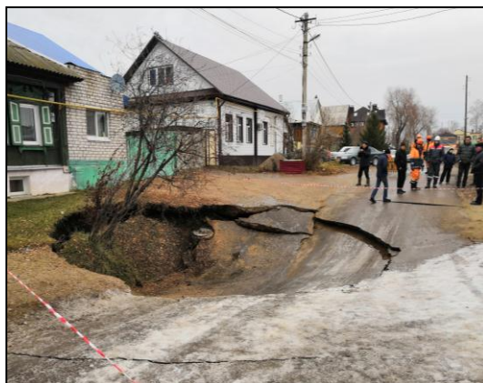
Figure 4 Karst failure in Ufa, st. Bolotnaya, d. 7. 19.11.2018. Photo A.I. Smirnova
