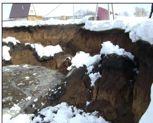
Figure 2 Karst failure in s. Novokulevo. 12.03.2017. Photo O.V. Sadykova
