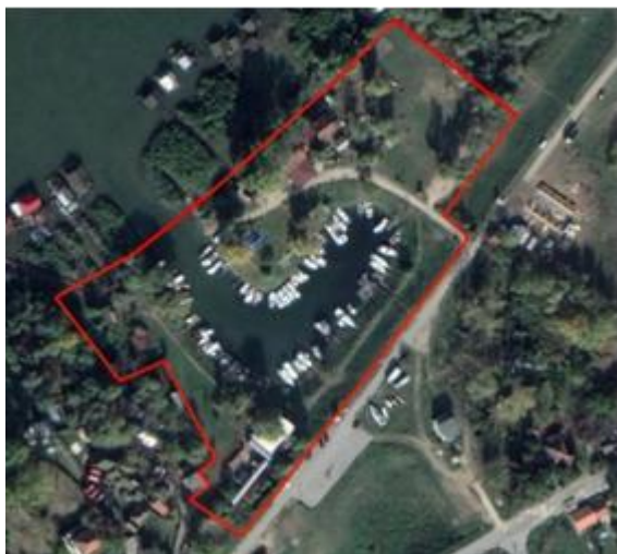
Figure 2 Orthophoto image of the researched area
